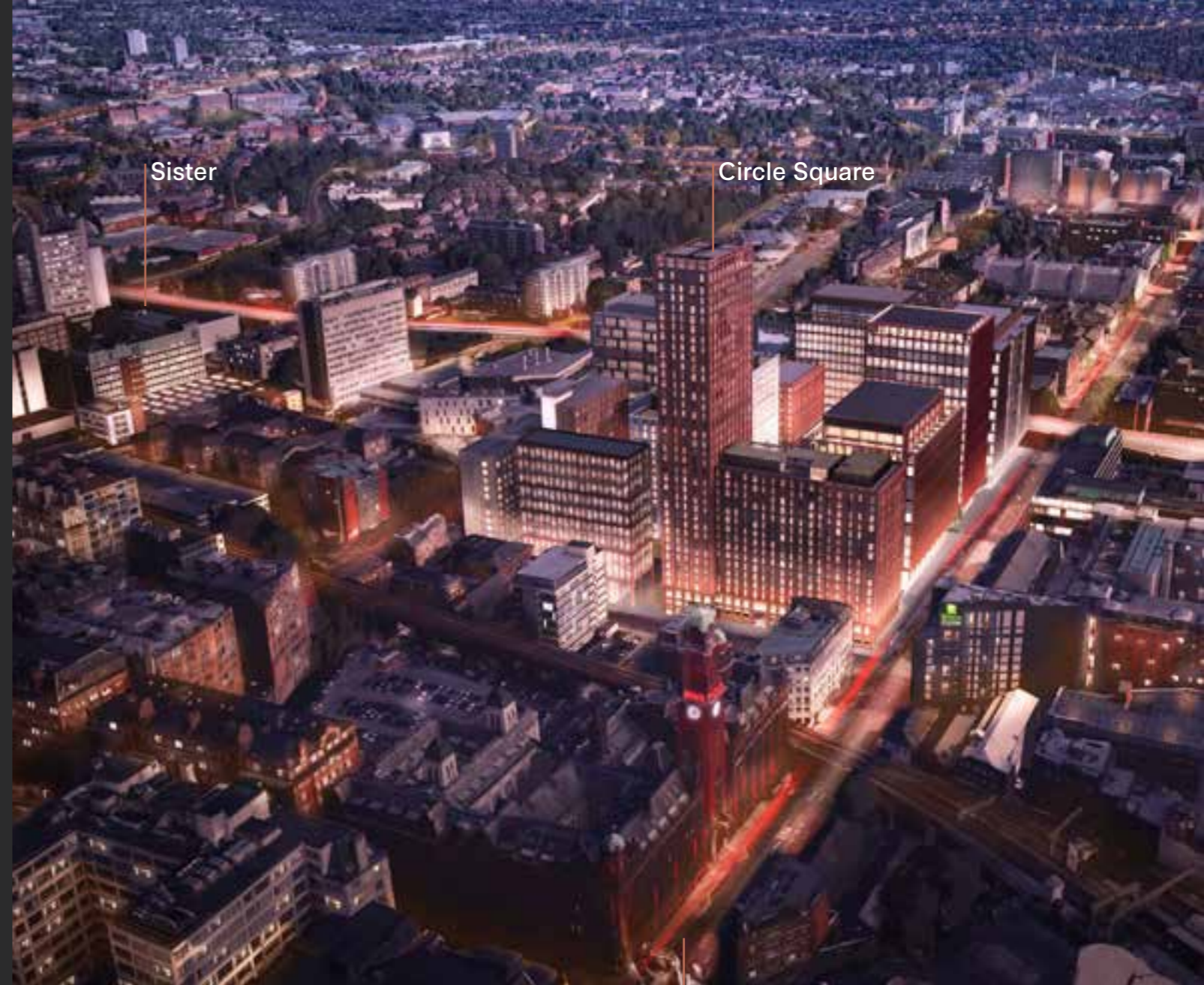
Oxford Road Corridor
